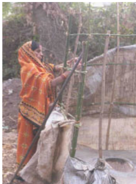
Building your first latrine superstructure
