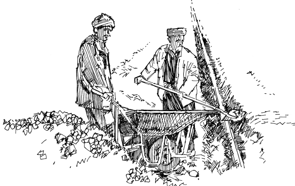
Backfilling
